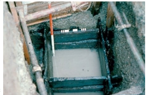
Lining 3 and 4 still left.
